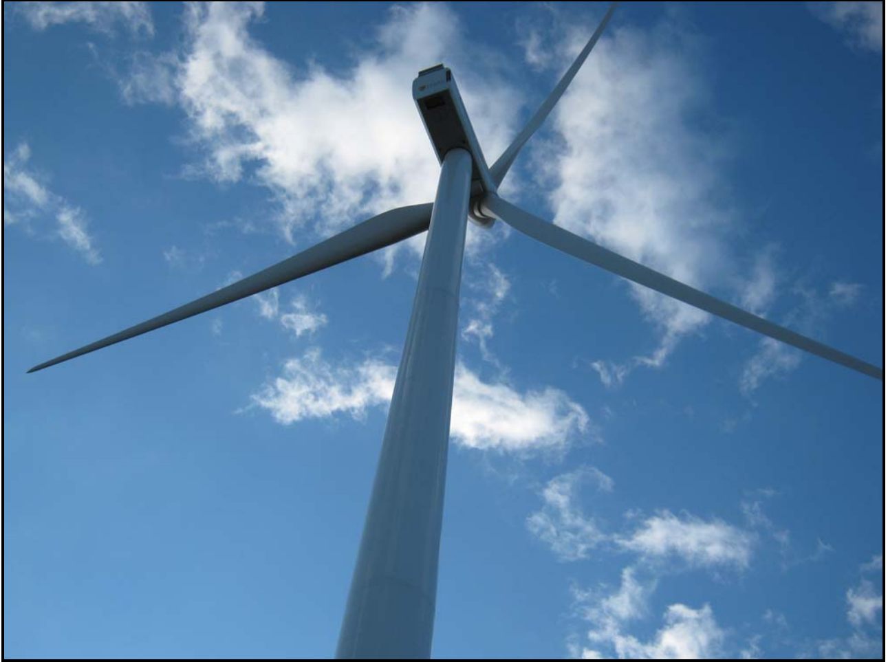
View of the UD-Gamesa wind turbine from the base of the tower.
